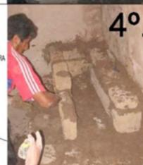
5. RECUBRIMIENTO INTERIOR DE LAS CAJAS CON MEZCLA A BASE DE: BARRO, VIDRIO CHANCADO, ESTIÉRCOL Y TUNA. ESPESOR: 3 cm.
